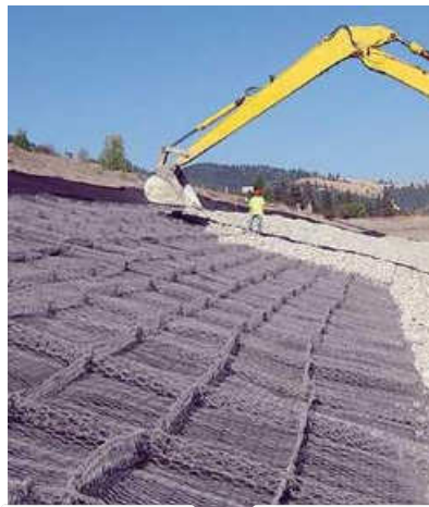
Soil erosion control
